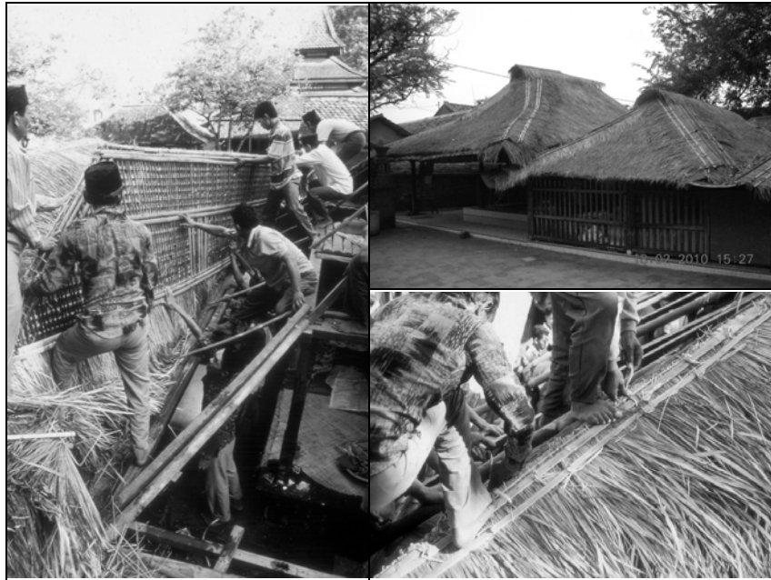
Figure 1. the Memayu festival in 2002 detaching the old roof (left), and assembling the new roof of the custodian building (right bottom and top). Photo: the author and courtesy of Murtiyoso.
