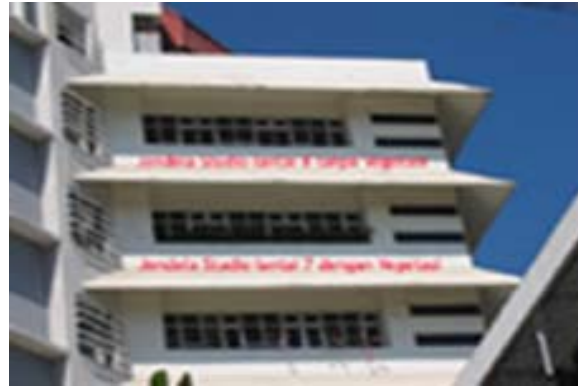
Figure 4. Window façade of the 7 th and 8 th floor studios
