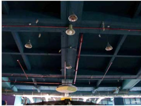
Figure 4 Lighting device and ceiling
