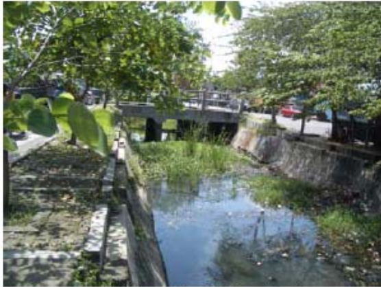
Existing Condition of the Urban Drainage in Raya Jemursari Street, Surabaya
