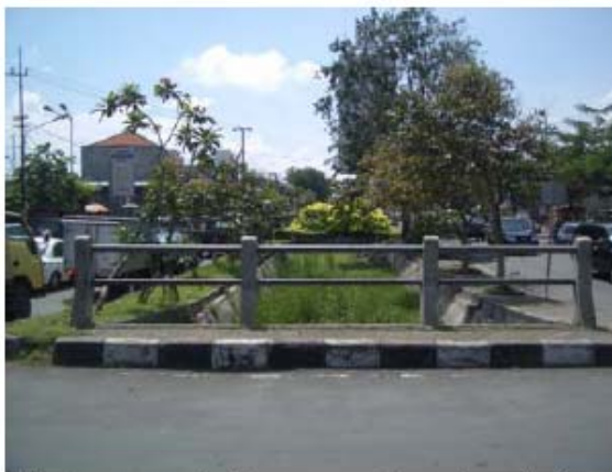
The turn over bridge a cross the urban drainage
