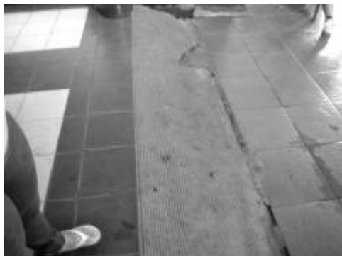
FIGURE 15. Inaccessible ramp and slippery floor surfaces
