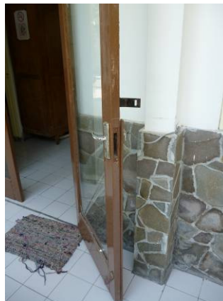
Figure .8. Dangerous door because it opened out to the pathway, causing many accidents to the blind students. And the sharp end of columns also that could harm Students.
