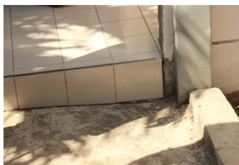
Figure 11. The harmful stair in the pathway end.
