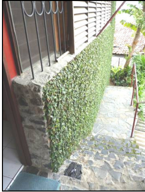
Figure 12. Bearing Wall from natural stone
