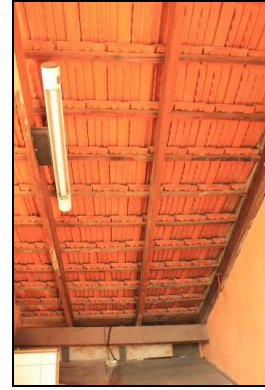
Figure 13. Construction of The Roof consisted of rafters, batten and tile
