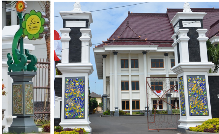
Image 13. Implementation of batik lokcan motif on column, gate, signed, and flower pots in the Regent's office in Tuban and the public area in front of it (Photo: Author, 2013).
