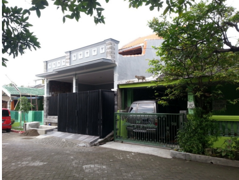
Fig. 2. Houses in Kemendung Indah Residence with full-front roofing. The roofs exaggerates on to the street kerb side.
