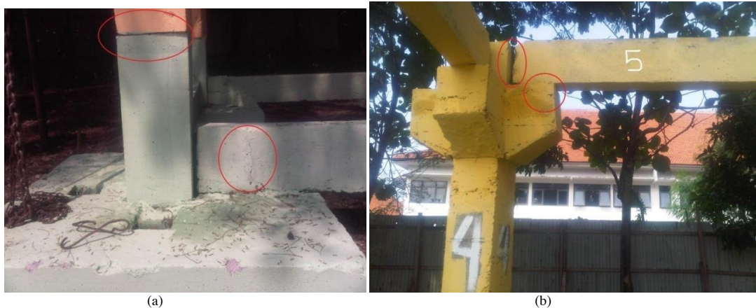
Fig. 6. The outcome after the 4 cm raise (a) crack in the tie beam connection and (b) deflection of the column.
