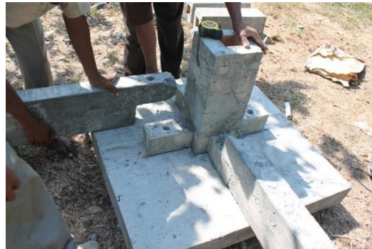
Fig. 3. Pedestal of type IV footings
