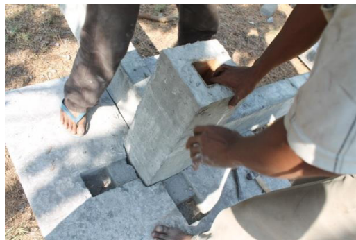
Fig. 2. Inserting the pedestal of type III footings
