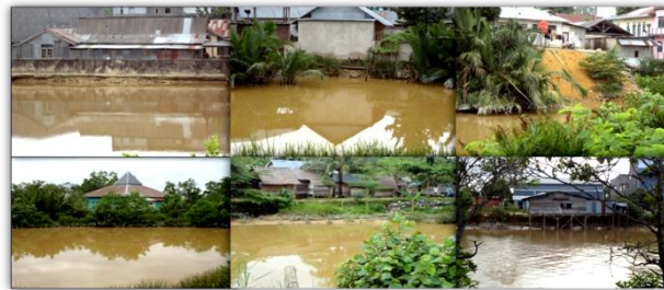
Figure 3. Old Retaining Wall, the critical condition of the settlement and places of worship, houses on the river and on the banks of the Wanggu River .
