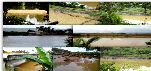
Figure 4. Sedimentation (Delta), Cracks embankment, empty stone masonry that needs repair, Dikes need strengthening towards erosion, sedimentation on the bridge abutments, Sedimentation and Erosion river banks of Wanggu .
