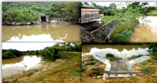
Figure 7. Box culverts, retaining walls, dikes and Wanggu River valve door.
