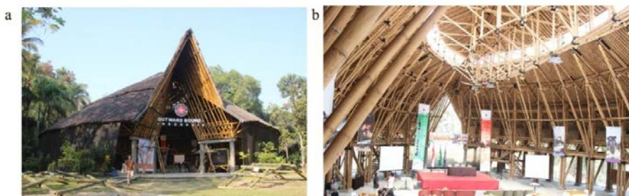
Fig. 3. OBI Great Hall (a) Building form; (b) Interior, show the structural system
