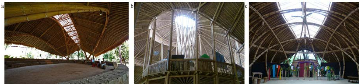
Fig. 6. Green School structure system; (a) Arches in main hall “Mepantigan”; (b) Surface structure in main building “The heart of Green School”; (c) Bamboo arches in classroom.
