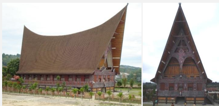
Figure 2: Gereja Katolik Inkulturatif Pangururan (GKIP) viewed from the side and front of the building
