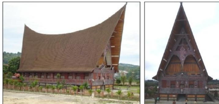
Figure 2. Gereja Katolik Inkulturatif Pangururan (GKIP) viewed from the side and front of the building (Photo: Author, 2015).
