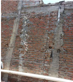
Fig. 11 Poor detailing at beam-column joint
