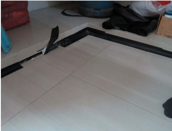
Fig. 5 Differential settlement of floor
