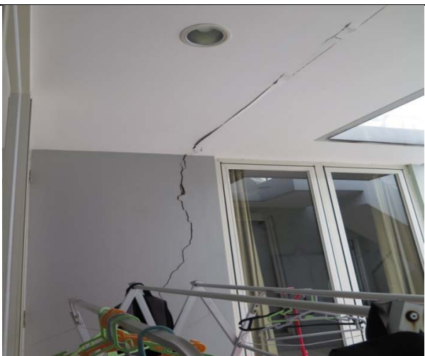
Fig. 9 Diagonal crack on the wall and ceiling
