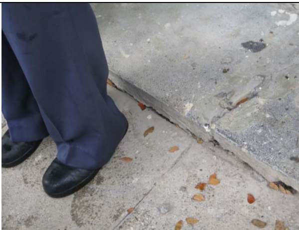
Fig. 7 Differential settlement of carport slab
