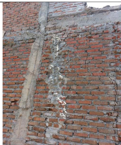
Fig. 10 Vertical cracks on the brick wall
