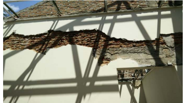
Fig. 12 Poor detailing of beam-column joint and horizontal cracks on the brick wall
