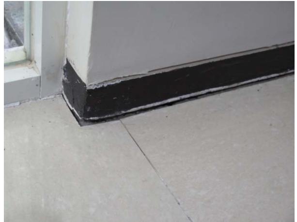
Fig. 6 Gap between floor and wall
