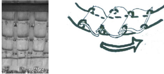
Figure 7. Photo of the detail roof coverings (Source: Maria I Hidayatun documentation, 2014).
