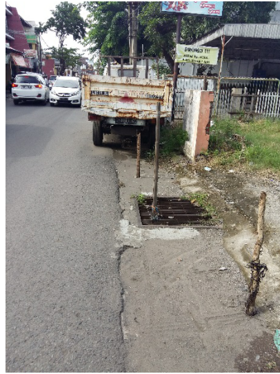
Fig. 4 The narrow and inaccessible pathway, the vehicle parking and vulnerable gratings causing the difficulty to access for all users.
