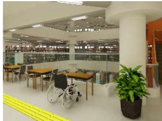
Figure 29. The Railing in 7th Floor with 150cm height
