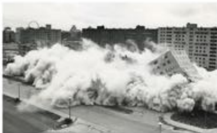
Gambar 3. 10 Penghancuran Kawasan Pruitt-Igoe (sumber : https://www.archdaily.com/870685/la5-classics-pruit-igoe-housing-project-minoru-yamasaki-st-louis-usa-modernism )
