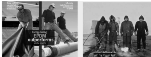
Figure 3: Applying Single-ply Rubber Membrane Roofing. (EPDM)
