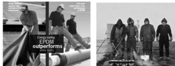
Figure 5. Applying Single-ply Rubber Membrane Roofing. (EPDM)
