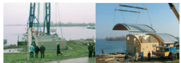
Fig.9. Delivery through water (Floating Houses IJburg)
