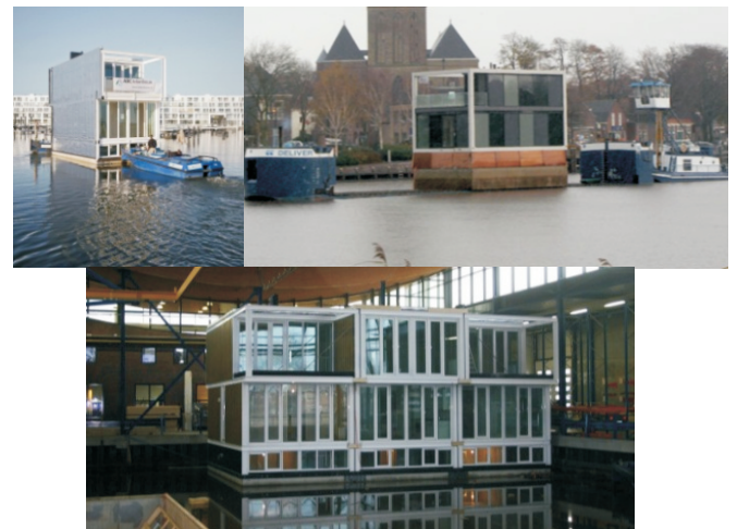
Fig.9. Delivery through water (Floating Houses IJburg)
