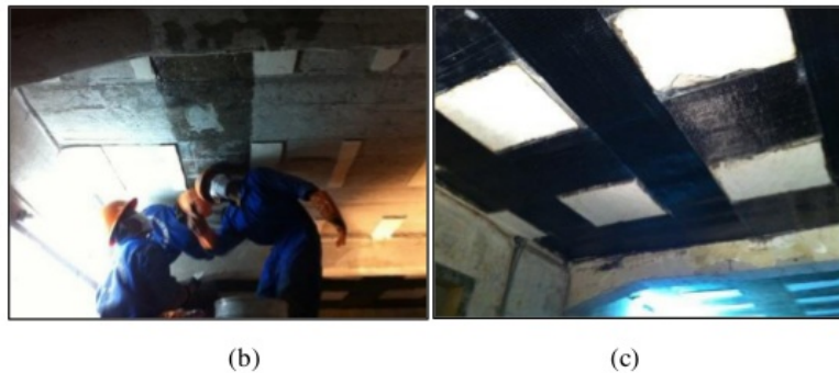
Fig. 3. (a) bottom slab strengthening; (b) beam strengthening; (c) installing fiberwrap on the slab.
