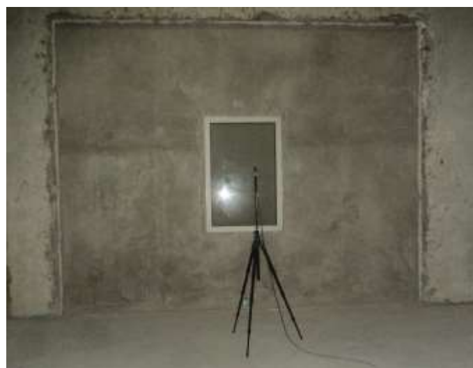
Fig. 2. Front view of composite wall specimen.
