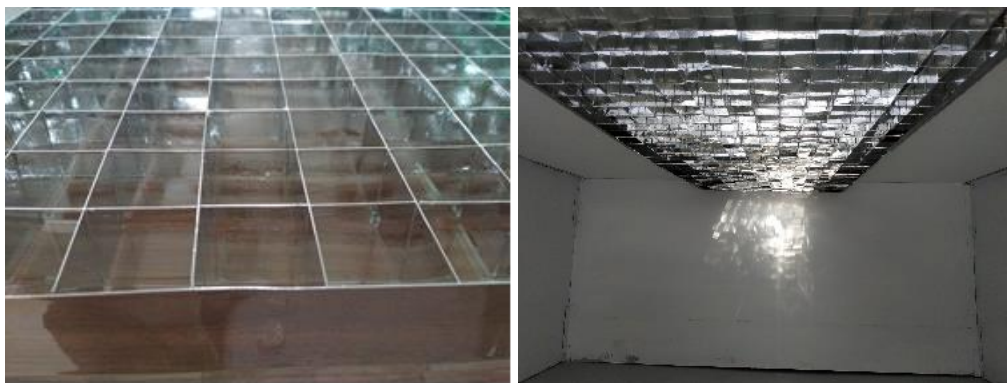
Figure 4. Chromed Egg-crate Reflector Panel at Horizontal Light Pipe's opening distribution.
