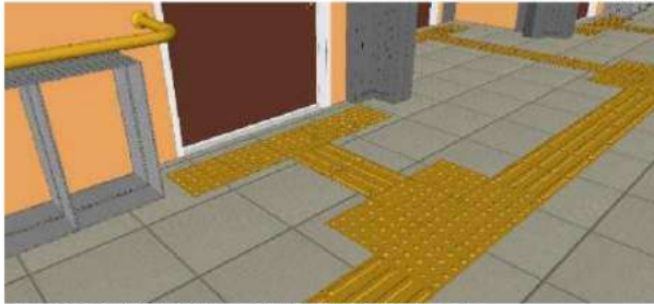
Figure 123 Detail of guiding path in the ideal school corridor.
