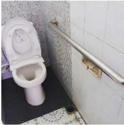
Figure 96 Construction of adaptive toilet, with sitting toilet, anti-slip flooring and railing.
