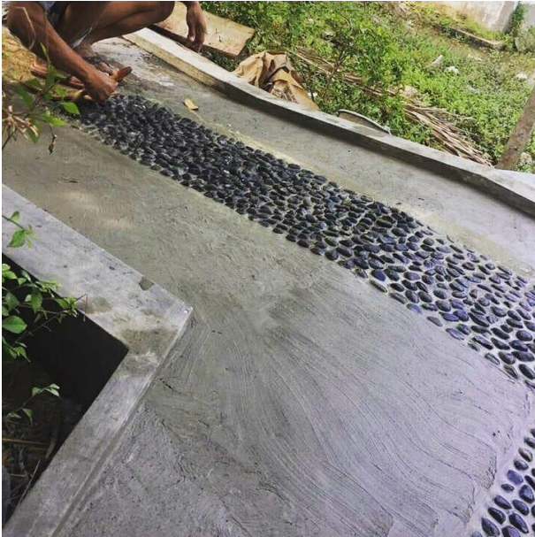
Figure 94 Construction of ramp and simple-rock-material-guiding path.
