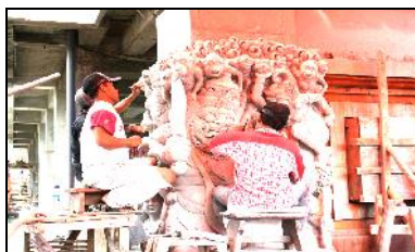
Fig. 8. Two undagi are working on the ornamentation of a building (Personal documentation, 2005).
