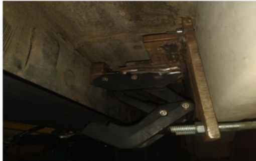
Figure 3. Installation of a footstep on the chassis.
