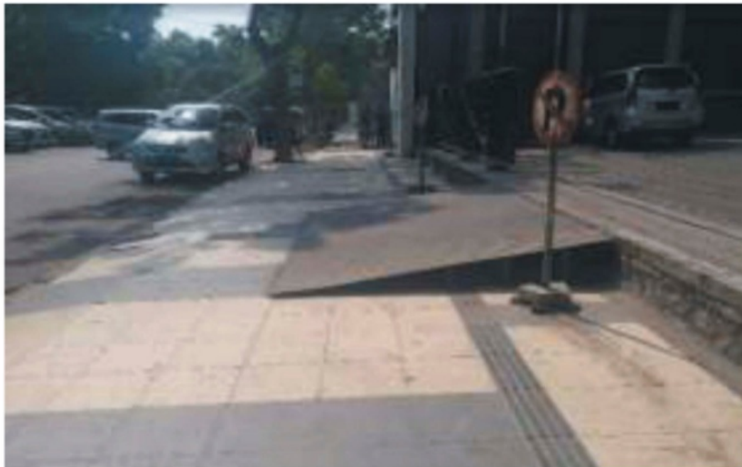
Figure 2. A snapshot of a non-accessible segment of pavements due to obstructions, a non-standard coloured and non-embossed guiding blocks of Surabaya's pavements.
