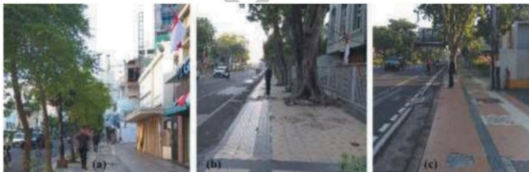
Figure 5. Typical pavements in the study (a) the Siola segment (the most improved pavement; 5 m width); (b) the Bambu runcing segment (4 m width); (c) the Darmo segment (2.5 m width).
