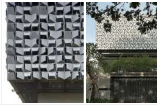
Figure 14. Block system on façade Source: https://www.archdaily.com/787057
