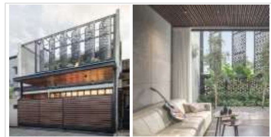
Figure 3. Fully ventilated system facade Source: https://www.archdaily.com/941186/
