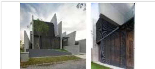
Figure 16. Natural material (bamboo) of façade Source: https://www.archdaily.com/109391
