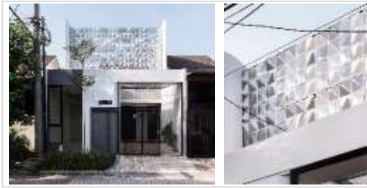
Figure 9. Perforated pattern and façade form Source: https://www.archdaily.com/951495
