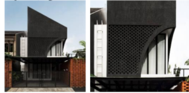
Figure 2. Semi ventilated secondary facade
