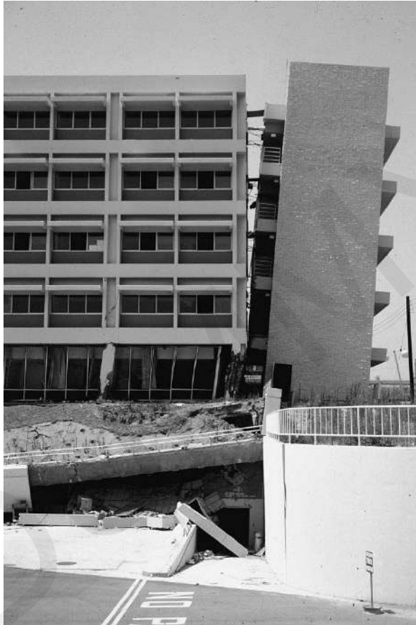
Gambar 29a. Olive View Hospital, San Fernando, California Tower Tangga Wing C Miring Karena Pounding
