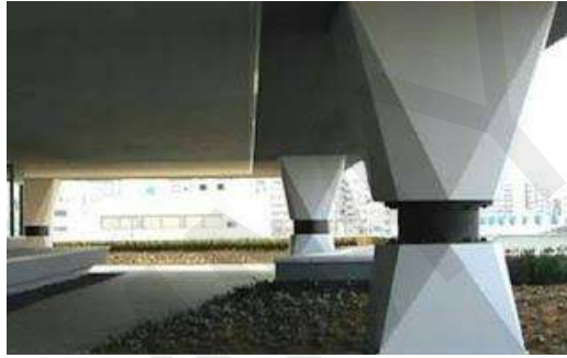
Gambar 151. Detail Base-Isolation
