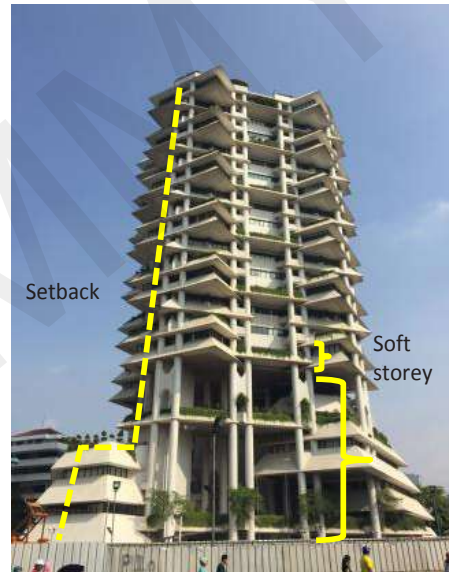
Gambar 140b. Intiland Tower
