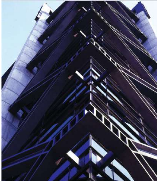
Gambar 147. Detail Bracing CEC Tower Taipei
