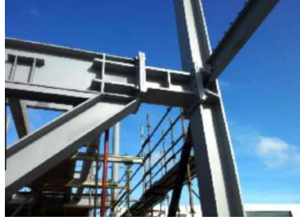
Gambar 83c. Removable Link Tepi https://www.buildmagazine.org.nz/index.php/articles/show/steely-performers , diunduh Juli 2021
