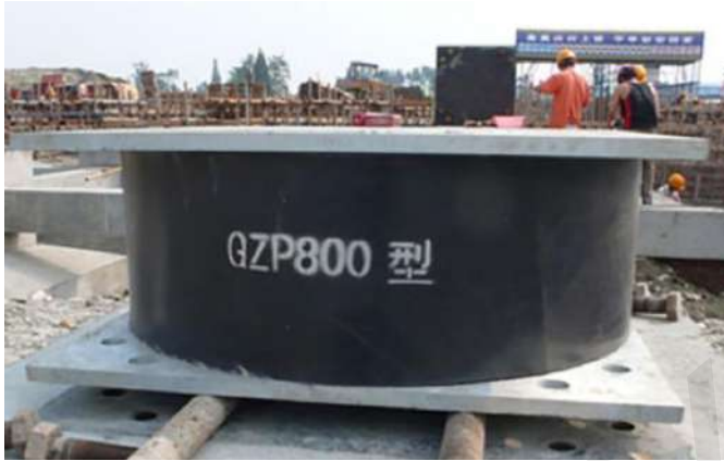
Gambar 89a. Laminated Rubber Bearing Base-Isolation
