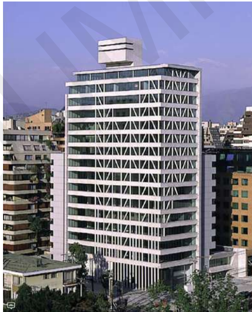
Gambar 137a. Manantiales Building Sudut Barat Daya
