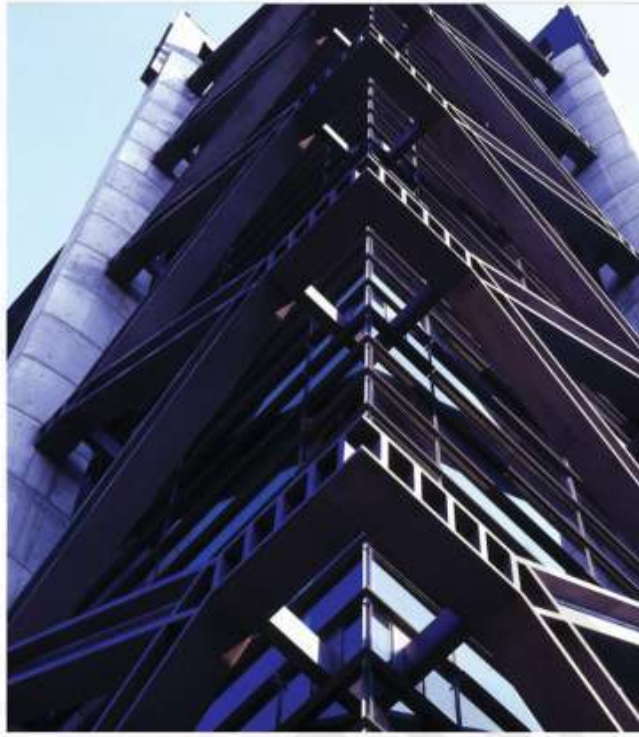
Gambar 147. Detail Bracing CEC Tower Taipei
