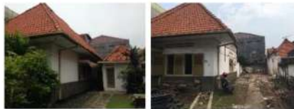
Figure 4. Before (left) and after (right) demolition.
