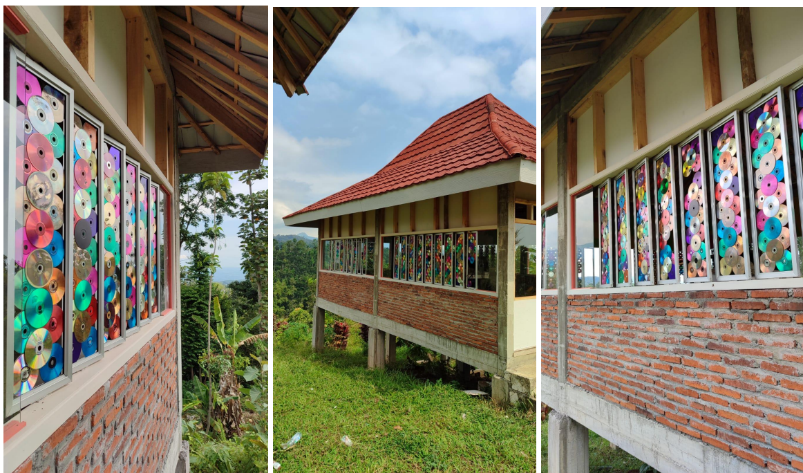
Gambar 3. The application of kinetic facade panel from recycled compact disc in the Tourism Hall - from exterior
