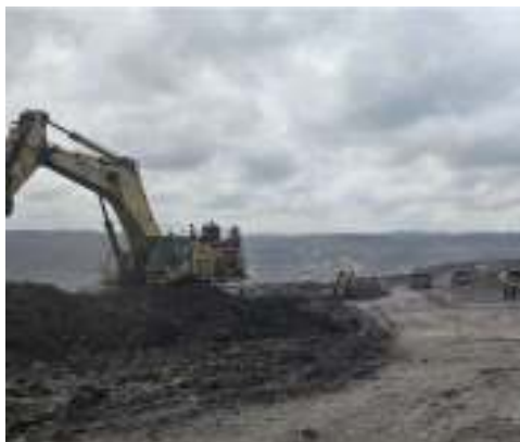
Gambar 6. Proses pembersihan sisa material ( spoil ) di tepi jalan
