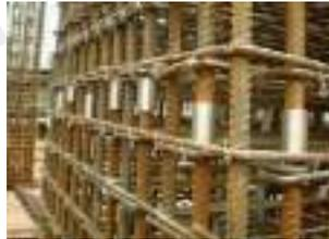
**Gambar 14.91** Sambungan Tulangan *Mechanical-Splice*
