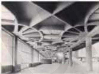
**Gambar 15.38** Struktur Lantai *Ribbed-Slab* Berpola Garis Isostatik Palace of Labor
