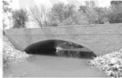
**Gambar 13.5** Barrel Vault Beton Betulang
