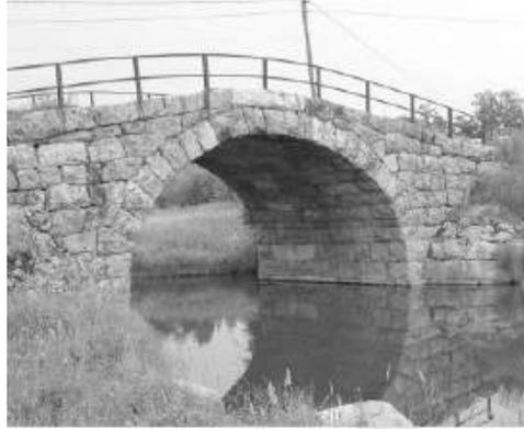
**Gambar 13.3** Barrel Vault Batu
