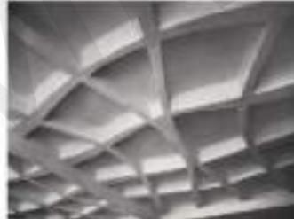
**Gambar 15.39** Struktur Lantai *Ribbed-Slab* Berpola Garis Isostatik Large Sports Palace
