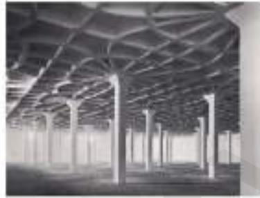
**Gambar 15.37b** Struktur Lantai *Ribbed-Slab* Berpola Garis Isostatik, Gatti Wood Factory
