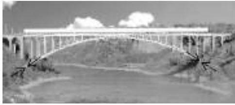
**Gambar 2.8 Form-Active Parabola Tekan**
