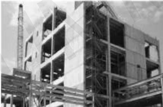
**Gambar 8.13b** *Frame - Shear Wall*
