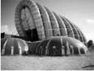
**Gambar 10.10** Struktur Membran *Air-Inflated* Tanpa Kover Eksternal
