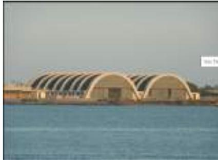
**Gambar 13.21** *Barrel Shell* Pendek
