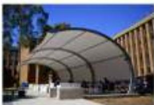
**Gambar 14.66** Kantilever Lengkung Pipa Baja
