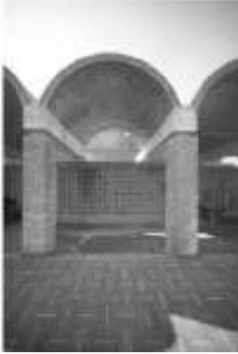
**Gambar 13.2** Barrel Vault Bata
