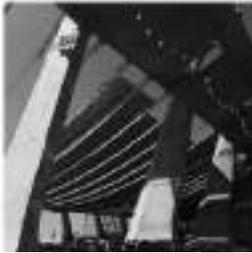
**Gambar 9.7c** Pemasangan Panel Atap Beton Pracetak Dulles International Airport
