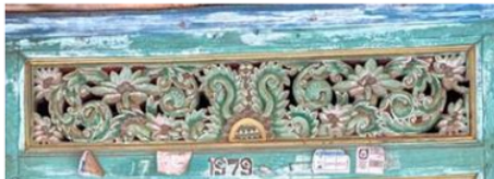
Figure 5 Gebluk Ornaments with Openings for Airflow Entry Source: Author, 2023
