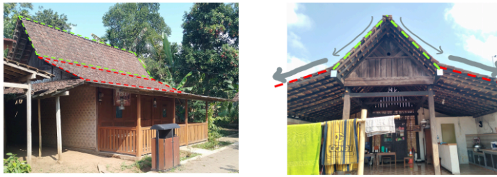
Figure 8. The two segments of the Tikel Balung Roof Source: Author, 2025
