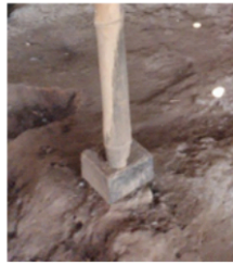
Figure 3. The connection between ubeg and sopak stone Source: Author, 2021
