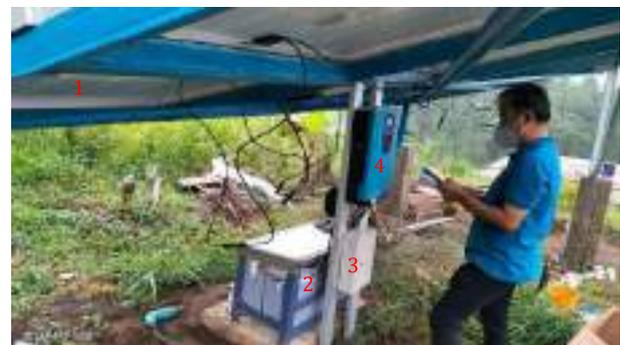
Keterangan: 1 = Solar panel; 2= Baterai; 3 = MCB dan kotak MCB; 4 = Inverter
