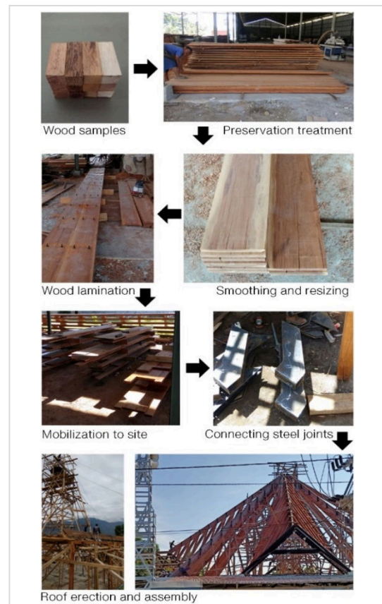
Figure 16. Wood sampling to roof structure erection process
