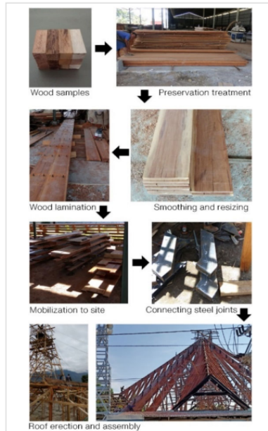
Figure 16. Wood sampling to roof structure erection process
