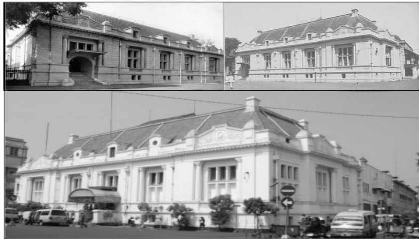
Figure 2. the buinding condition in c.1915 (top left), in 1922 (top right), and in 2009 (bottom). Source: KITLV (foto c.1915 and 1922)
