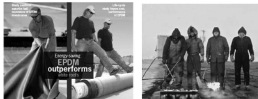
Figure 3: Applying Single-ply Rubber Membrane Roofing. (EPDM)
