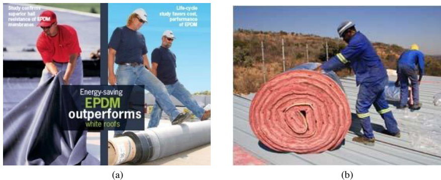
Fig. 3. (a) Roll of white EPDM membrane; (b) Roll of glasswool-aluminium foils outer roof insulation
