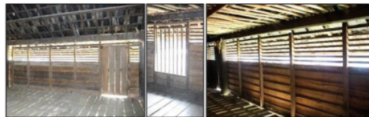
Figure 5. Doors, windows and lattices in the ceremonial room (Photo: Devina Faustine, 2016).
