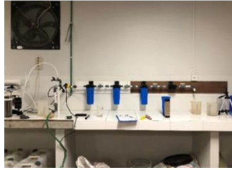
Filter Module Installations (b)
