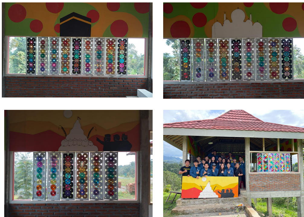
Figure 2. The application of kinetic facade panel from recycled compact disc in the Tourism Hall - from interior
