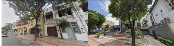
Figure 3.4 Building Facades Around Rajawali Street Google Street View, 2023
